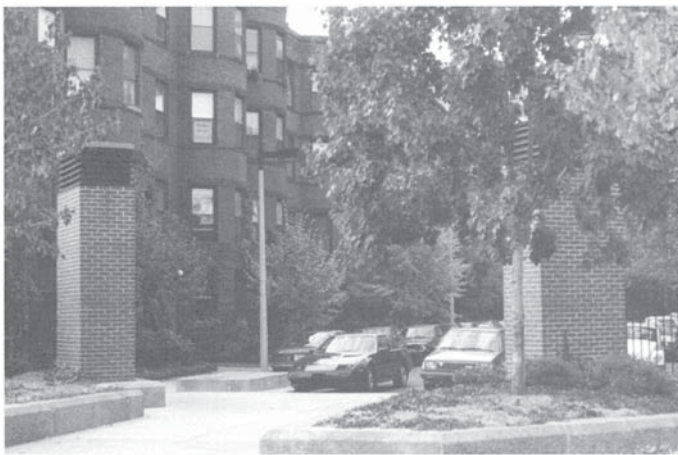
Fig. 3. Park gates are integrated with the pumping station ventilators on the Southwest Corridor.
